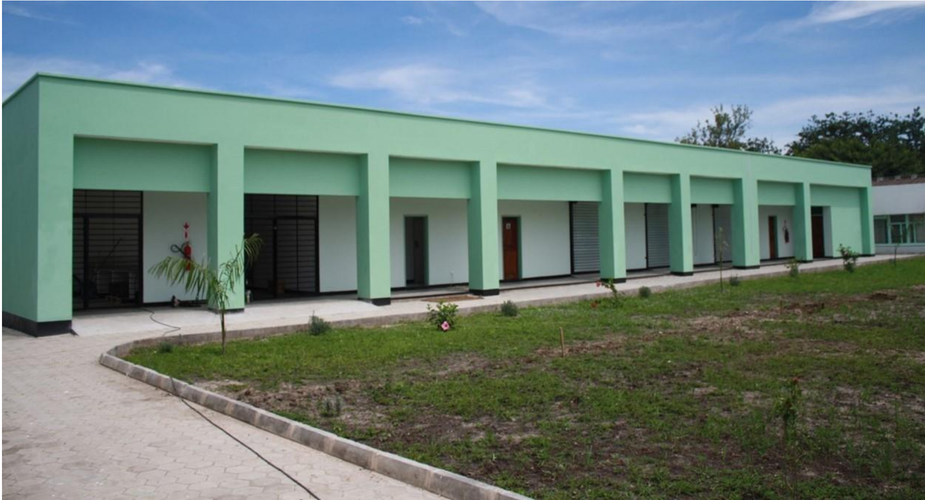
Maintenance Building – Side/Front View
